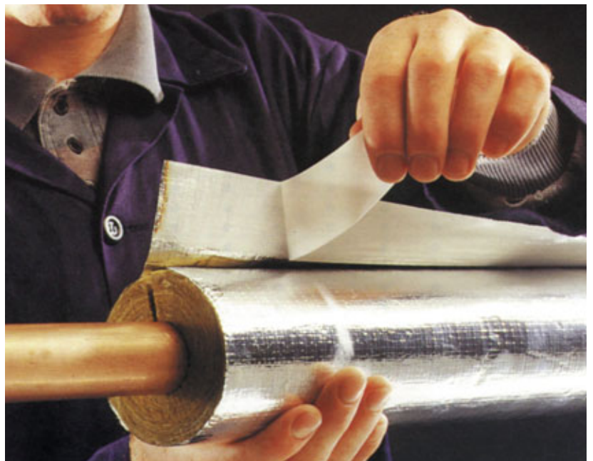
Fast installation of Rockwool Rocklap H&V Pipe Sections to copper pipes
